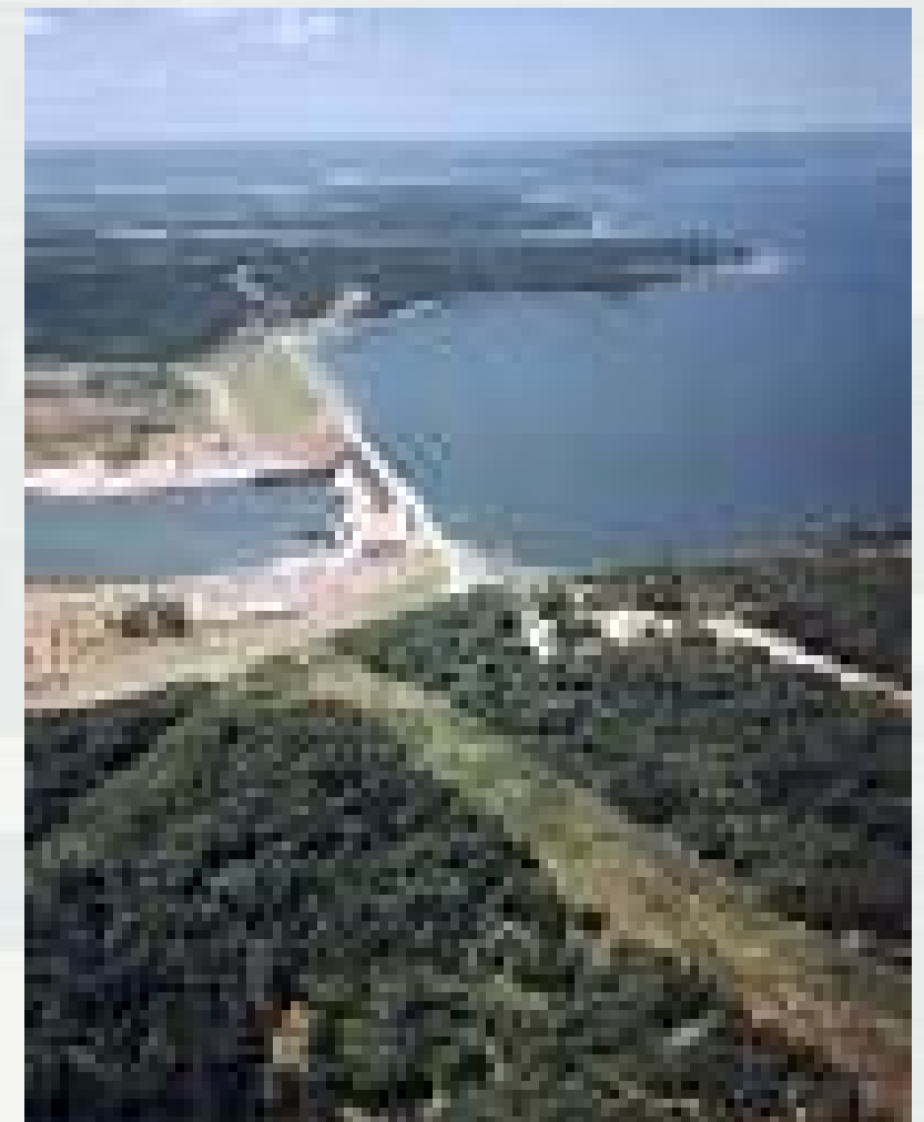
Eufaula Lake Dam site
